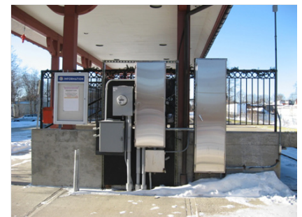
Automatic Snowmelt System on Platform
