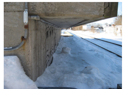
Close-up of Automatic Snowmelt System Piping
