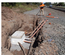
Replacement handhole for Berlin train station communication house
